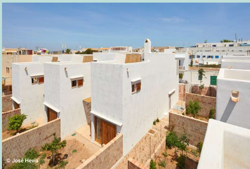
Figure 5.1 Posidonia project, Balearic Islands, Spain
