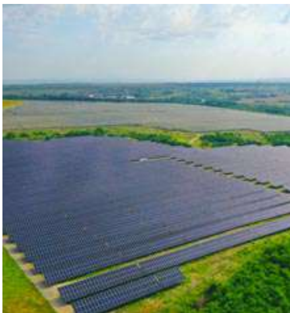
82 MW PV park installed in 2023 at a site of a former dump of opencast lignite mine, near the village of Mednikarovo, Bulgaria.
