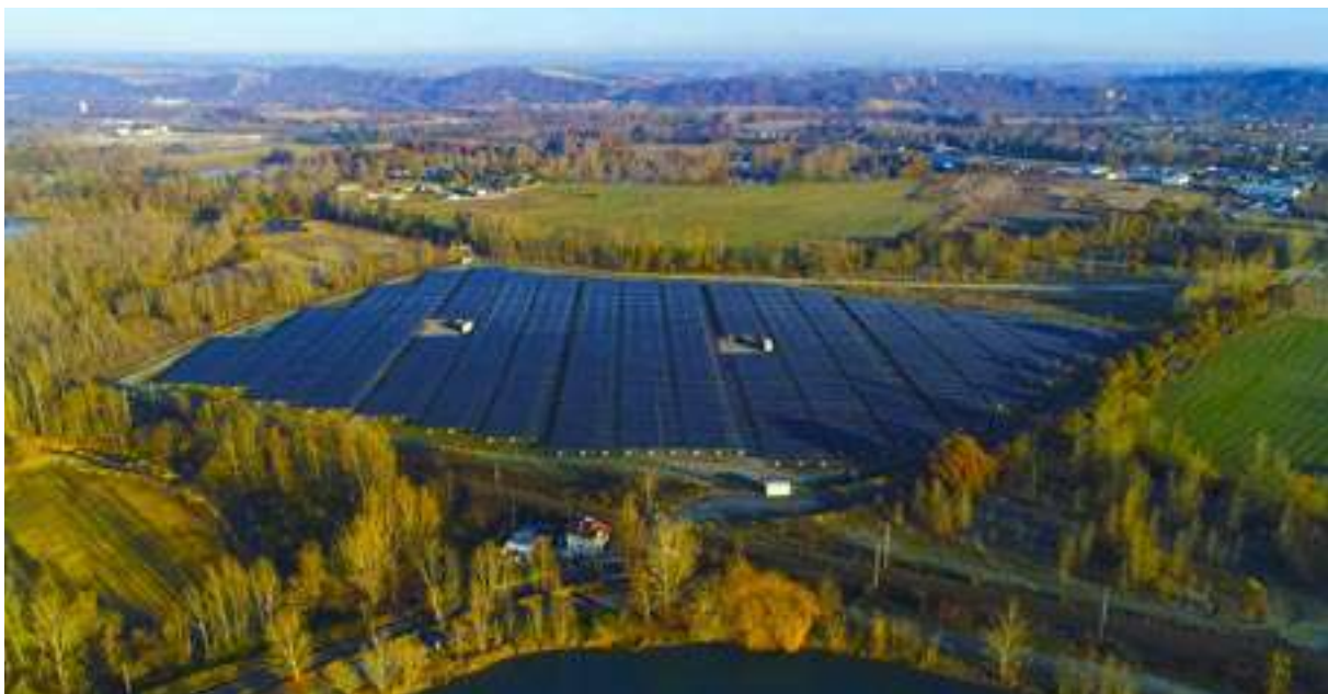
Solar park in Lavernose, 5 MW, located in a former gravel quarry.
