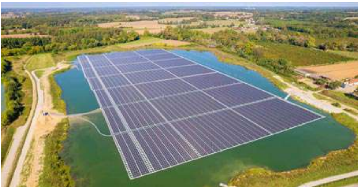
11 MW, Gouts, France.
