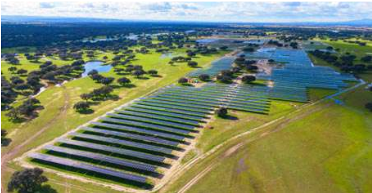
300 MW Talayuela solar park, Caceres, Spain.
