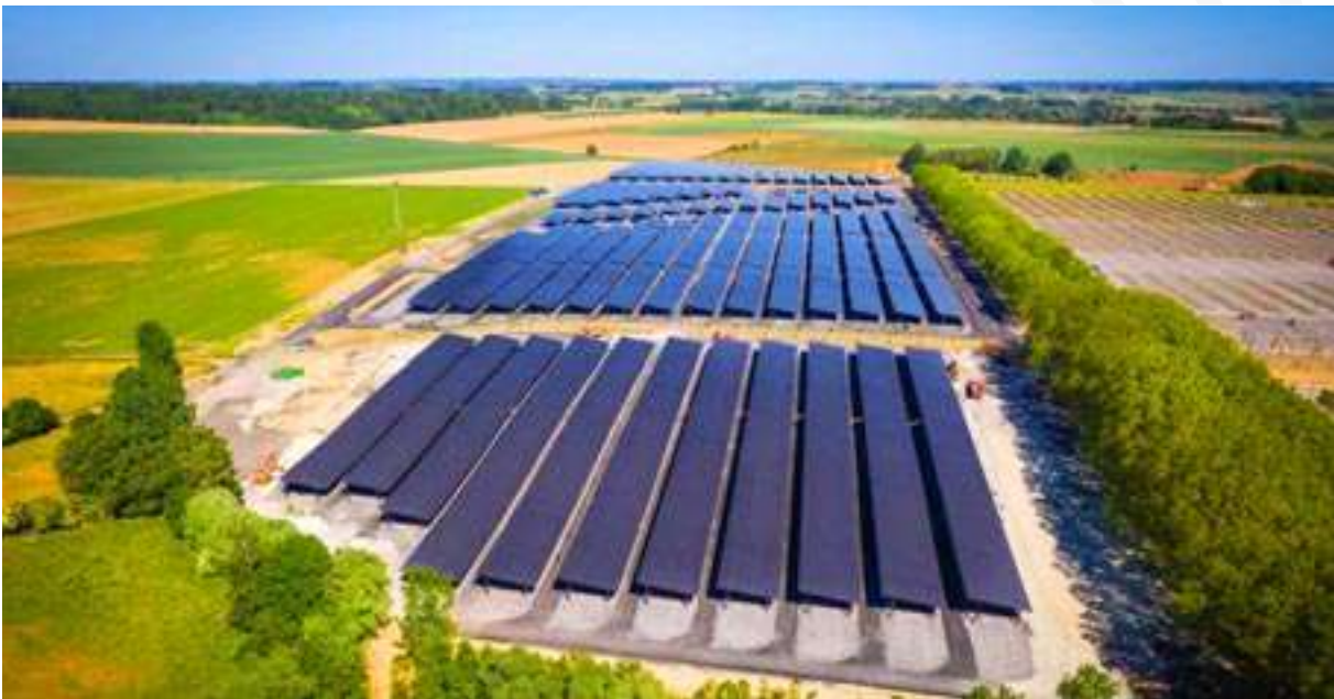
19.9 MW, Brugelette, Belgium.
