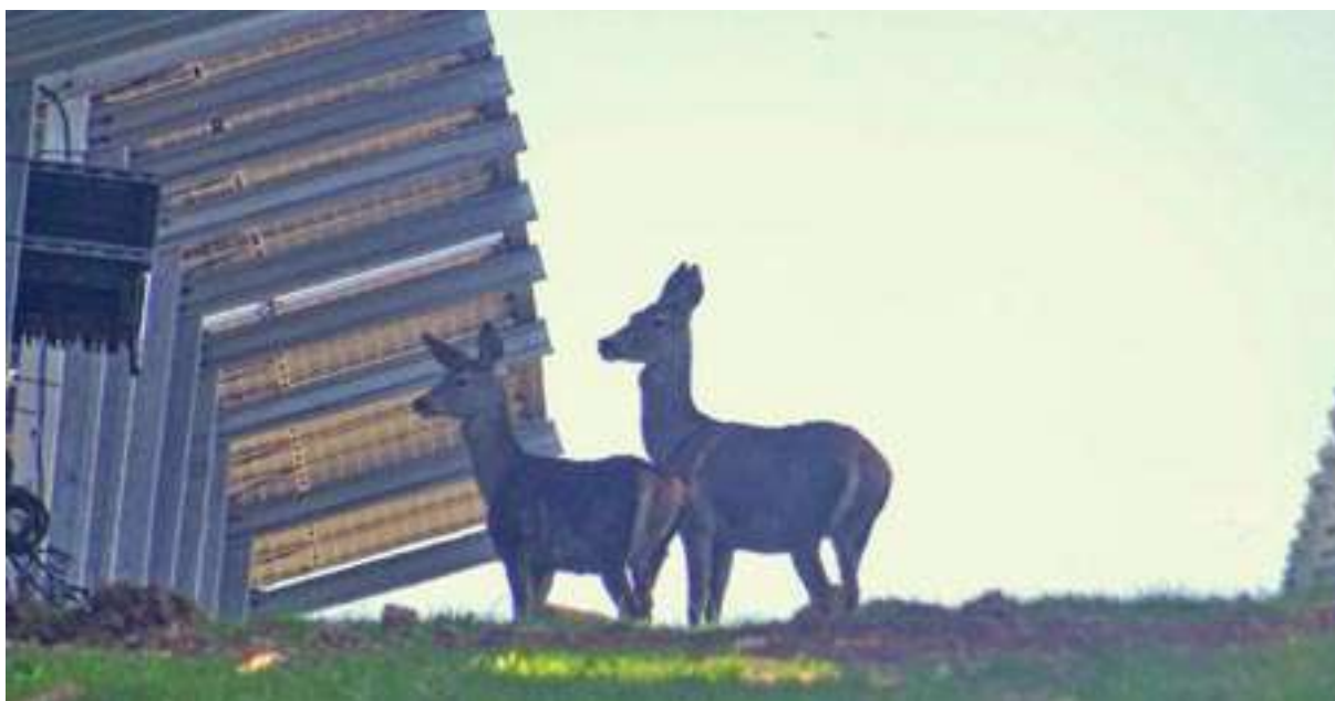
40 MW attached to a 3 MW / 9 MWh battery, Campo Arañuelo III in Almaraz, Cáceres.
